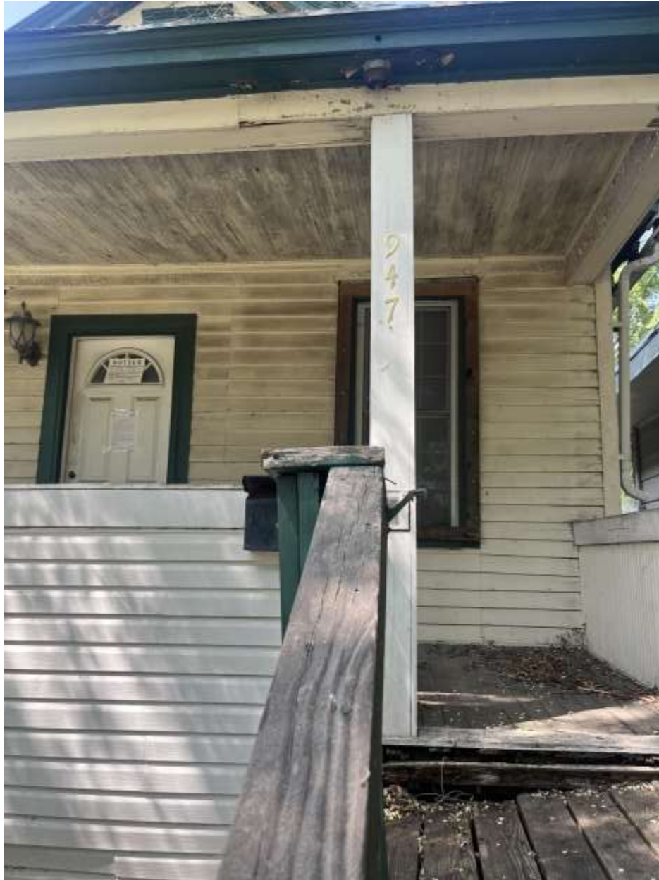
947 Fremont Ave.contractor photos 6-2-25
